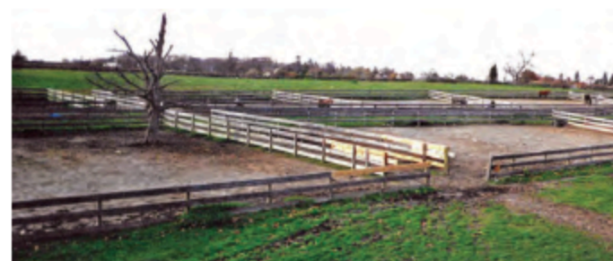
Paddock system under construction for horse turnout.
